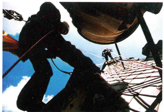
INDELEC technicians installing a LPS on a bell tower
