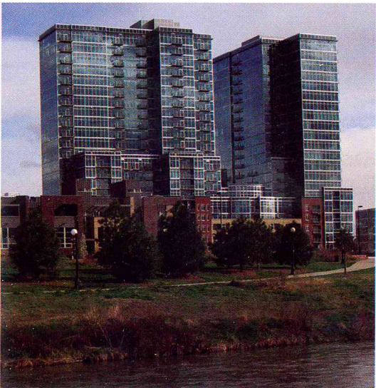
The Glass House condominium - Colorado - USA
