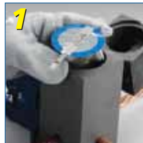
1 Insert CADWELD PLUS package into mould
