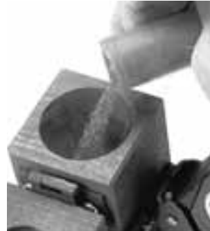
Step 3 Dump welding material and tap bottom of container to release starting material
